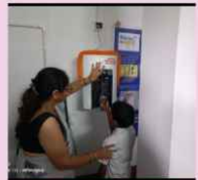
IWC ASANSOL GREATER SET UP OF WATER PURIFIER
